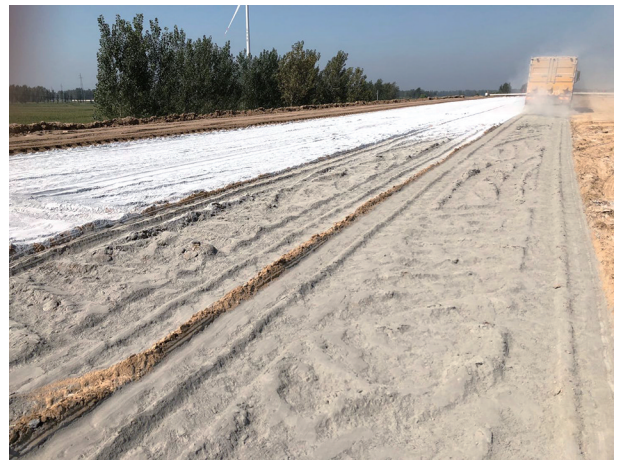
图 5 试验段改良剂与水泥对比 Fig. 5 Comparison of modifier and cement in the test section
